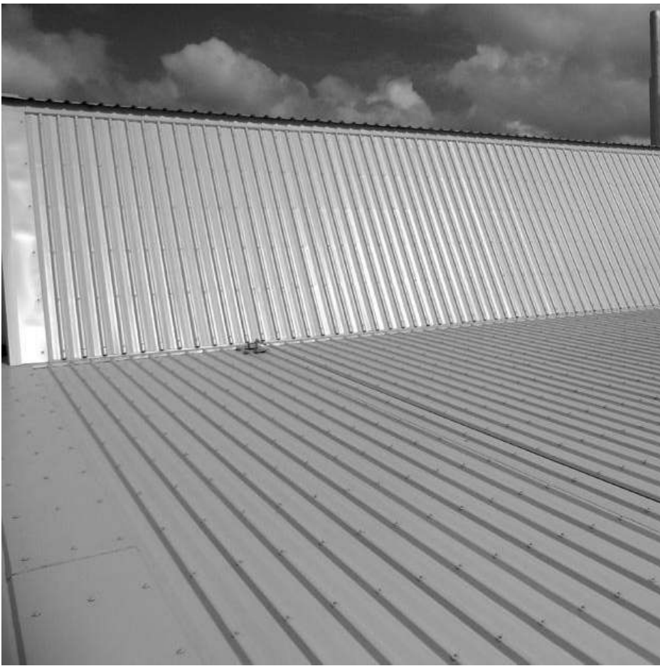
TRIM-DEK ROOF SHEETING - GREY - TO MATCH WALL CLADDING
